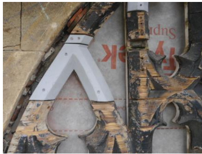
Repairs to St John, Banbury
